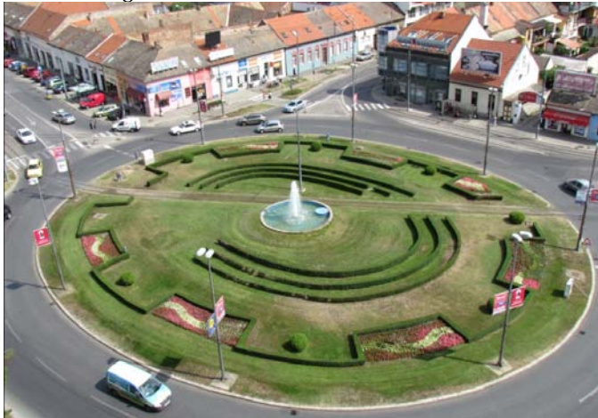
Figure 2 Two-lane roundabout „Đakovština“
