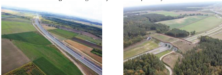
Figure 4 Fragments of S8 and S5 expressways in Poland
