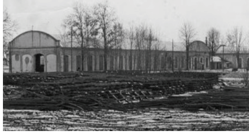
Image 3 Hemp plant Hungaria under construction (1905.)
