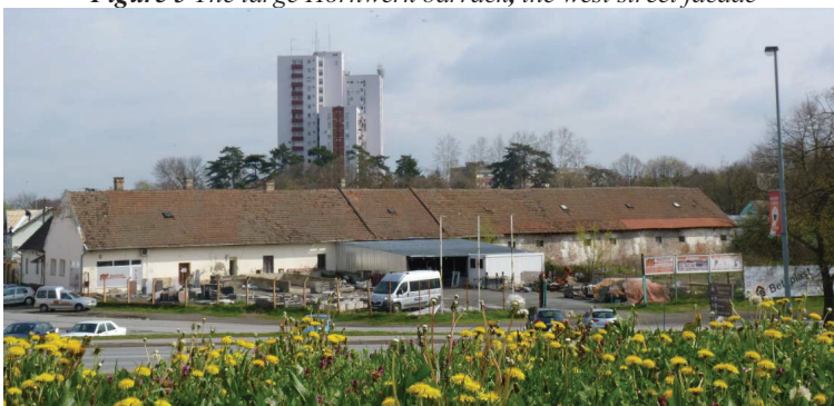
Figure 5 The large Hornwerk barrack, the west street facade
