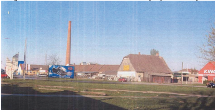
Figure 8 The small Hornwerk barrack with roof before it collapsed
