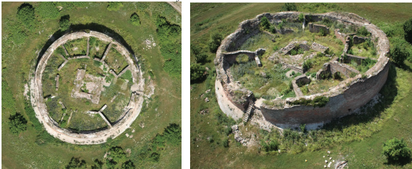
Picture 9 Korođvar fortress – documented with UAV
