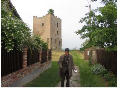
Picture 1 The Tower of Erdut 7
