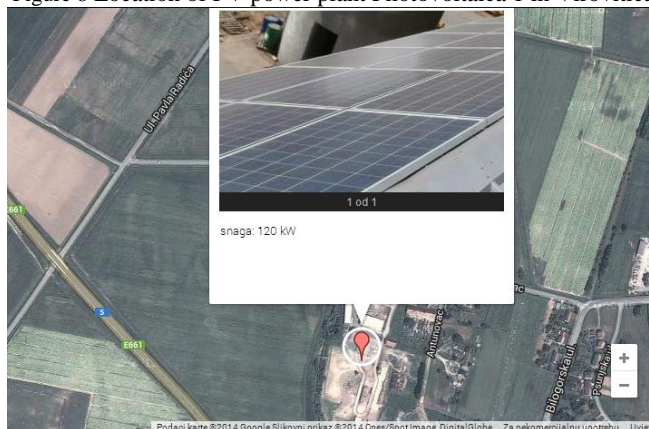
Figure 8 Location of PV power plant Photovoltaica 1 in Virovitica
